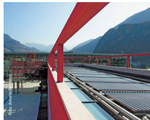
Main building of EURAC research in Bolzano
